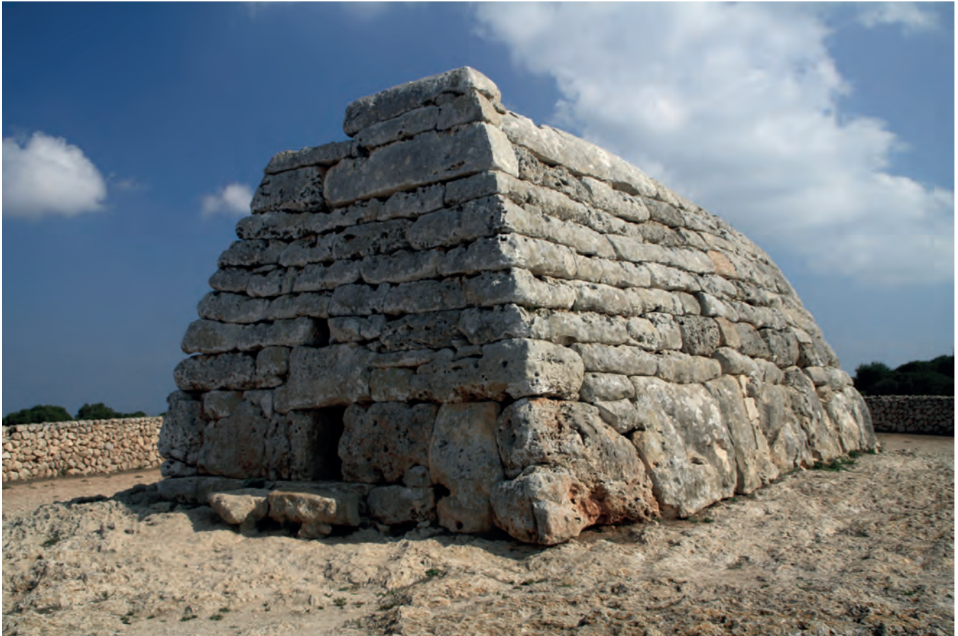
FIGURE 5. Naveta in Tudons. This is a burial naveta in the shape of an inverted ship built with the cyclopean technique during the Bronze Age and located within the township of Ciutadella (Menorca).
