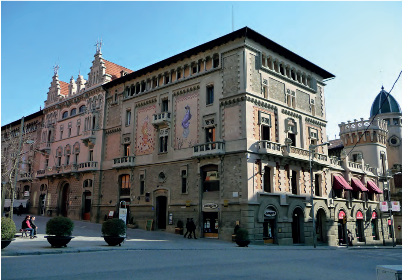
FIGURE 1. Façade of the Athenaeum of Vic, formerly Casa Comella. It is an Art Nouveau construction built in 1896 with mediaeval influence. In 1899, the Athenaeum moved its headquarters to the Art Nouveau-style Casa Comella located next to Plaça del Mercadal.
